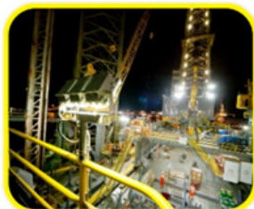
Petrol Process Factory
